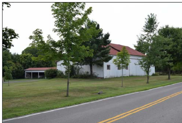
5927 Rings Rd, English barn, looking southwest
