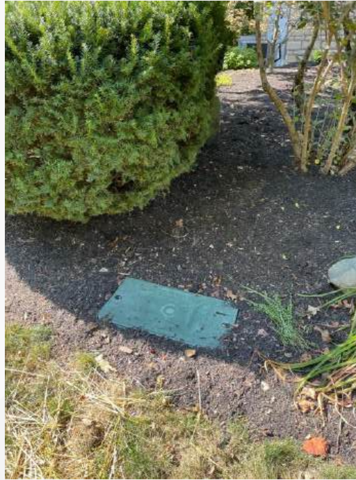
Final installed fiber optic pull boxes
