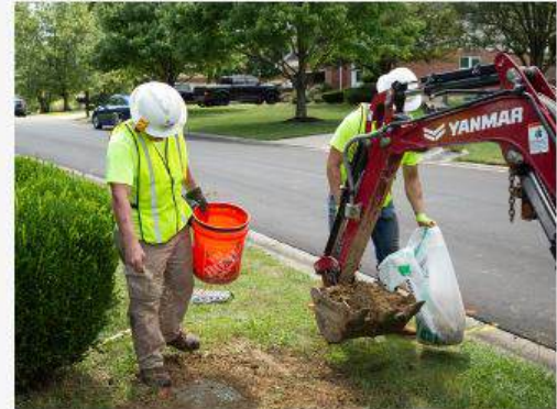
Placing seed for restoration
