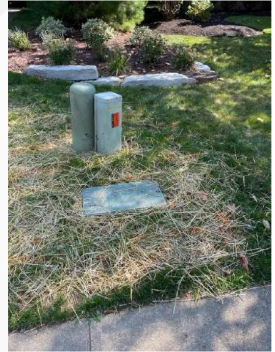
Final installed fiber optic pull boxes
