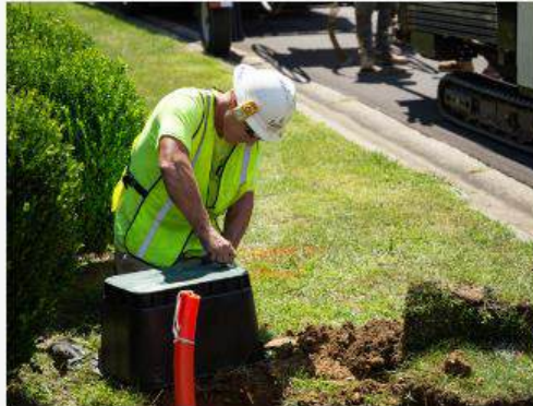
Placing pull box
