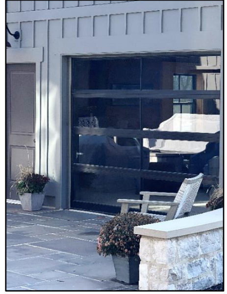
Aluminum Glass Doors with Windows 181 S High Street (Residential) New Construction Approved May, 2022
