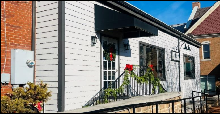
LP Siding (smooth texture) Modern Male Salon ( Commercial ) Landmark Property Approved September, 2021
