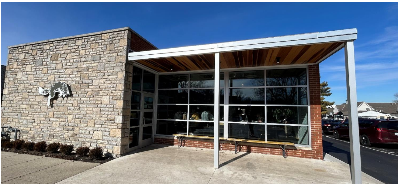
Adaptive Reuse, Fox in the Snow, 38 W. Bridge Street
