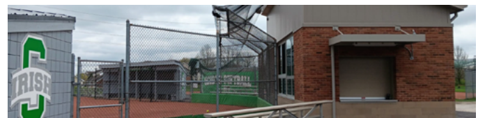
Dublin Scioto Softball Building, 4000 Hard Road
