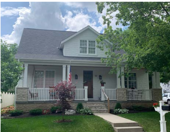
Finished foundation, 73 South Riverview Street
