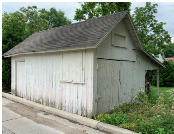
Historic outbuilding, 83 South Riverview Street
