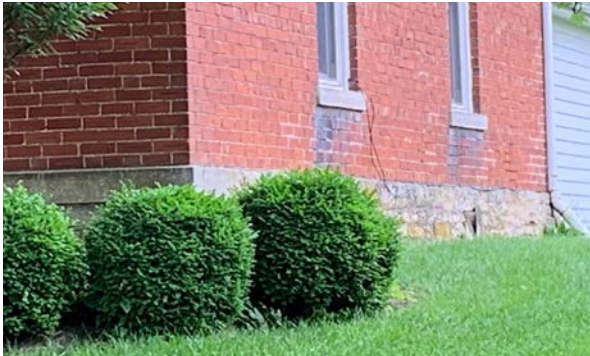
Original stone foundation, 167 South High Street
