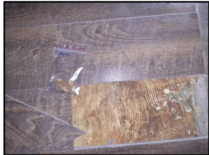
4 – HA 4 - Vinyl Floor Cover (Brown, Imitation Wood) with Backing (White)
