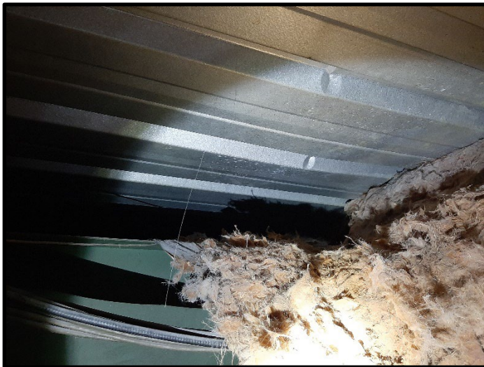
23 – View of a ceiling at top of the building
