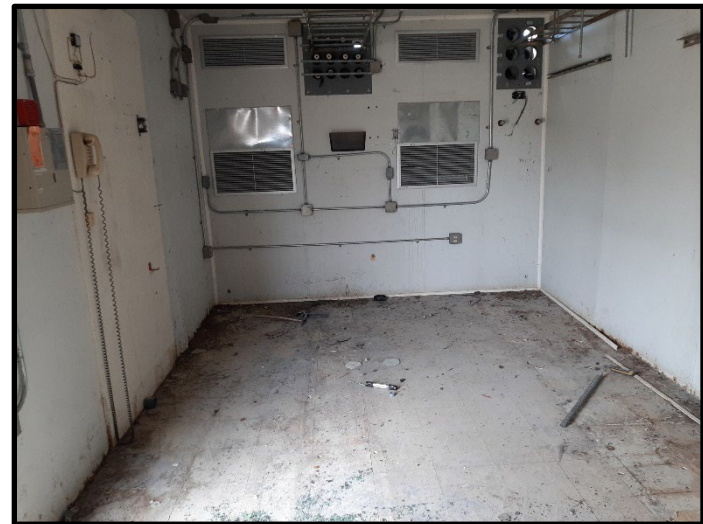
24 – View of inside of the telecommunications building
