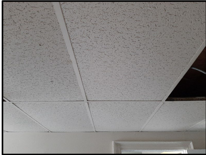
9 – HA 9 – Drop Ceiling Tile (Gray with White Surface, 2'x4')
