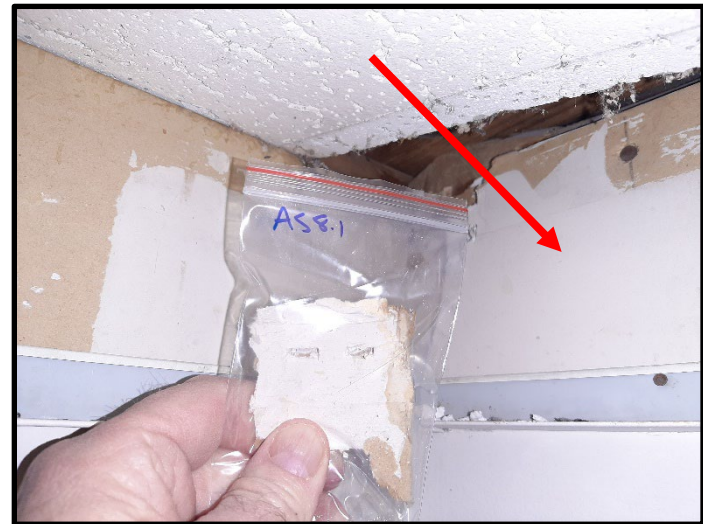
8 – HA 8 - Drywall (White) with Joint Compound (White)
