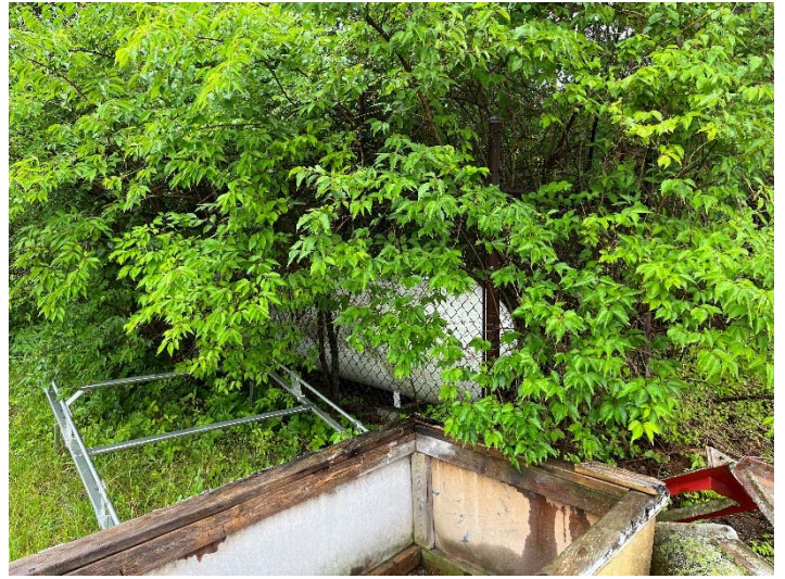
Figure 4. Natural Gas Tank
