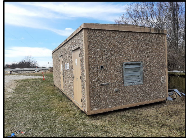
14 – View of the telecommunications building
