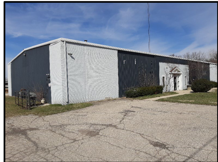
12 – View of the east and south sides of the building
