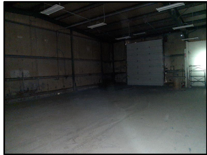
16 – View of Room 105
