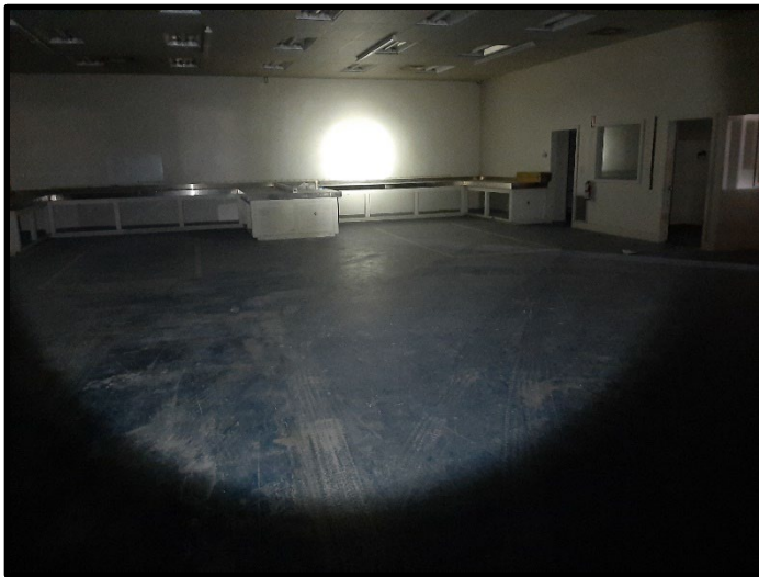
15 – View of Room 101
