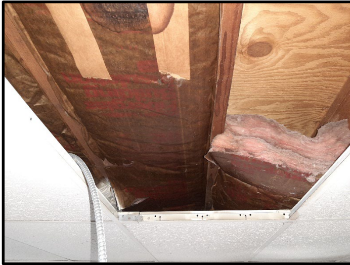
21 – View above ceiling tile in office area
