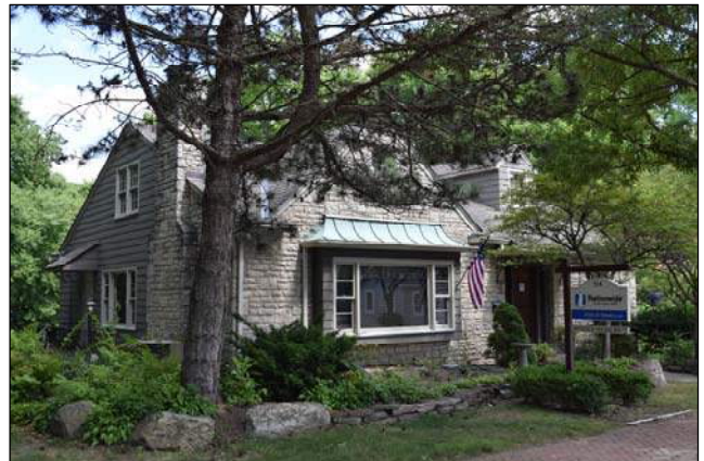
114 S High St, looking southeast
