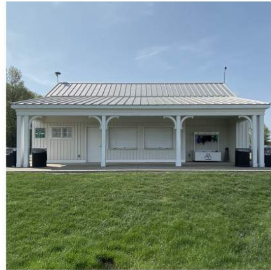
EXISTING NORTHWEST RESTROOMS
