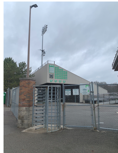
Existing View of Stadium and West Ticket Booth
