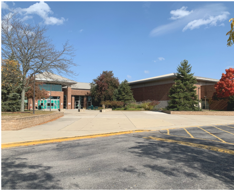
Existing Views of High School Building
