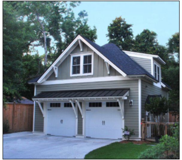
Rear Located, Front Accessed Garage w/ Carriage Doors & Transom Windows, Shed Roof Overhang & Decorative Brackets
