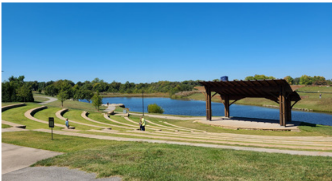
Amphitheater integrated adjacent to regional stormwater basin. Norton Commons--Louisville, KY
