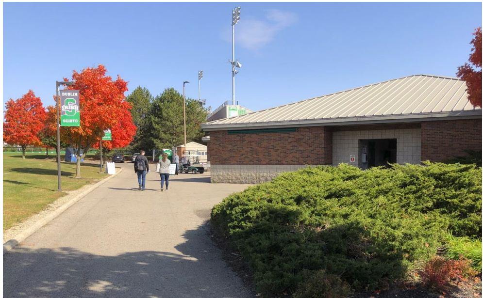
Above: Existing Stadium Concessions/Toilet Building (South of Stadium, One of Two)
