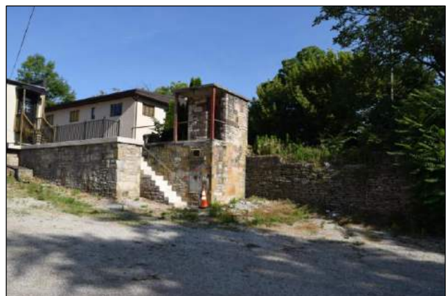
36-38 N High St, stone privy, looking northwest
