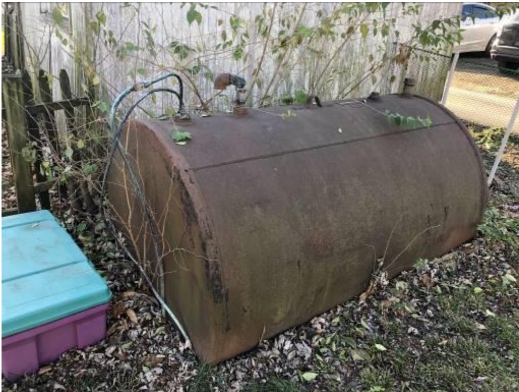
Photograph 2 – A heating oil tank remains in the southwest corner of the back yard and should be removed.
