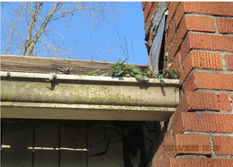
Photo 11 – View of improperly installed chimney flashing
