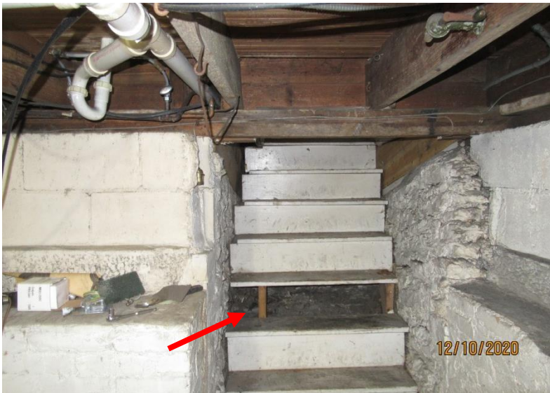
Photo 23 – View of basement entrance steps showing a missing riser face and no hand rails
