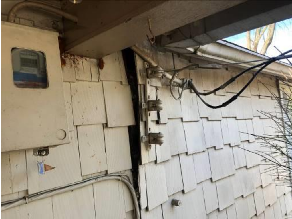
Photograph 5 – Secure the main electric service which is pulling loose from the front of the house.
