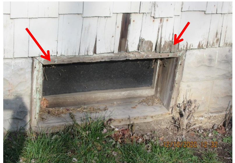
Photo 8 – View of basement window showing deteriorated siding and window frame
