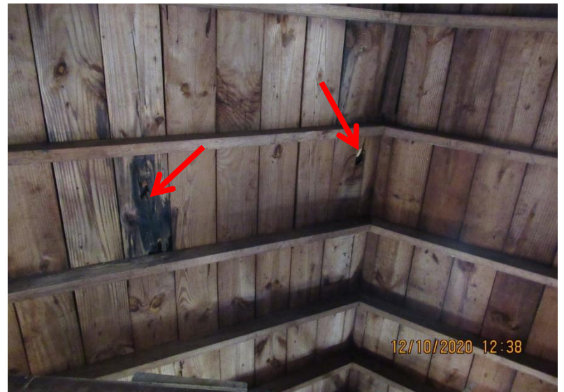
Photo 16 – Interior view of roof decking showing signs of water staining and holes in wood sheathing
