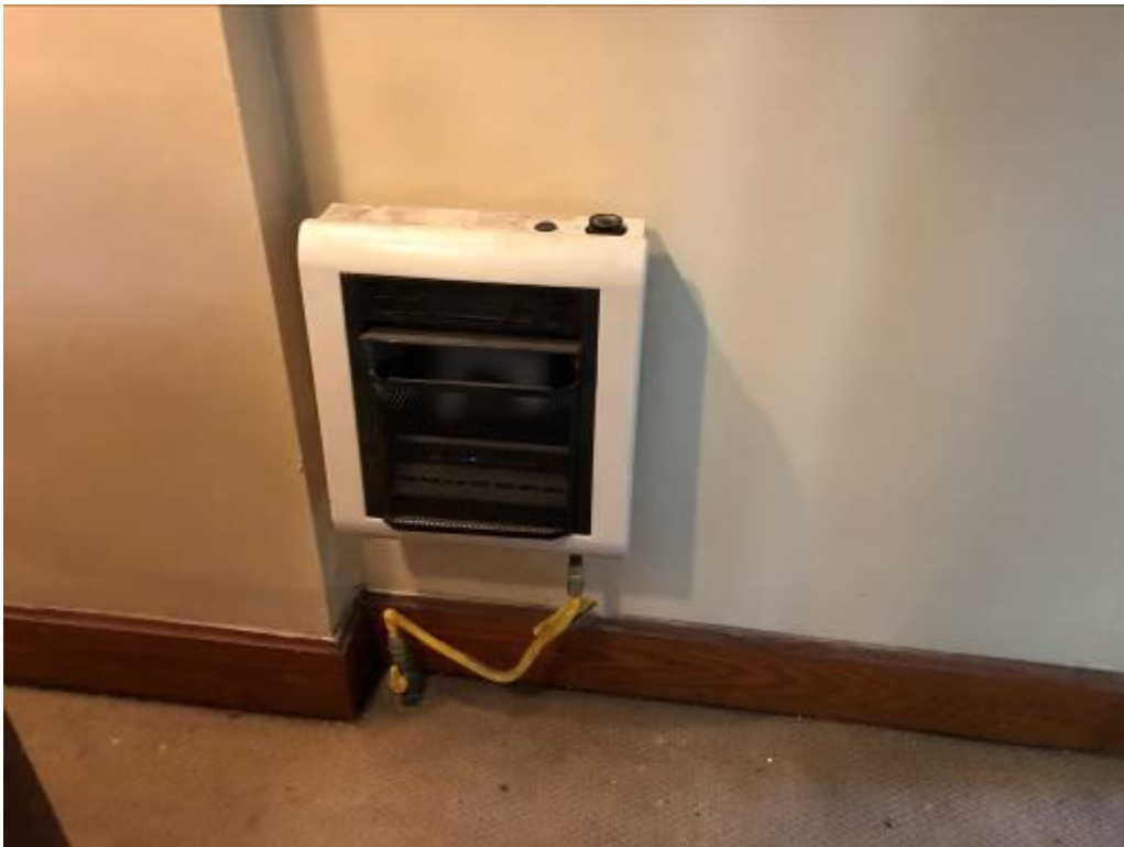
Photograph 4 – A gas fired heater in the rear hallway heats the northwest section of the house.
