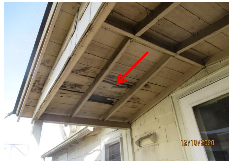
Photo 12 – View of the back porch roof decking showing signs of wood rot
