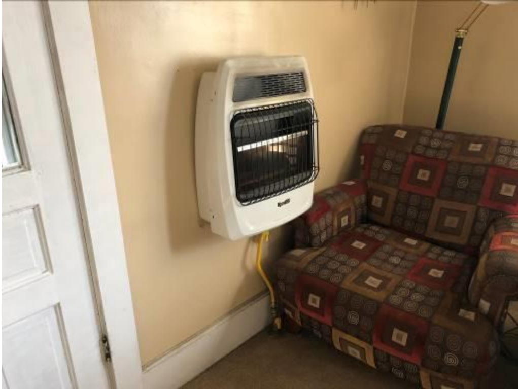
Photograph 3 – A gas fired wall heater by the front door heats the living room.
