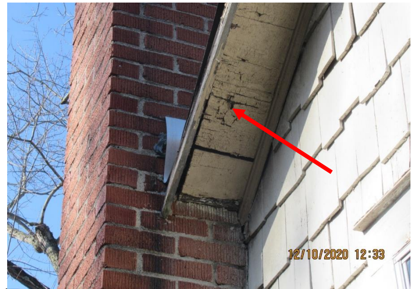
Photo 10 – View of deteriorated wood soffit panels
