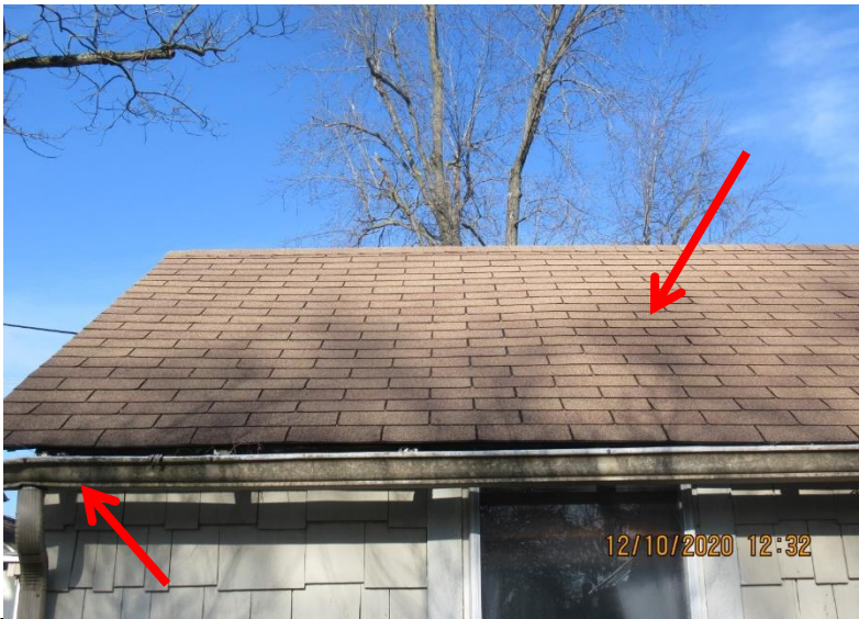
Photo 9 – View of residence shingle roof and deteriorated gutter
