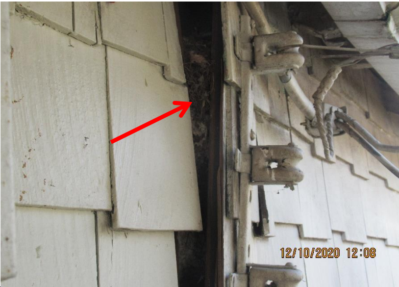
Photo 5 – Main electric line pulling siding off residence
