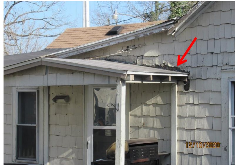
Photo 6 – View of deteriorated shakes on rear of residence
