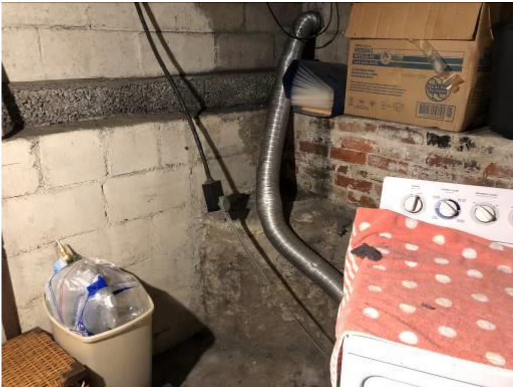
Photograph 6 – The electric dryer outlet is not property secured to the wall.
