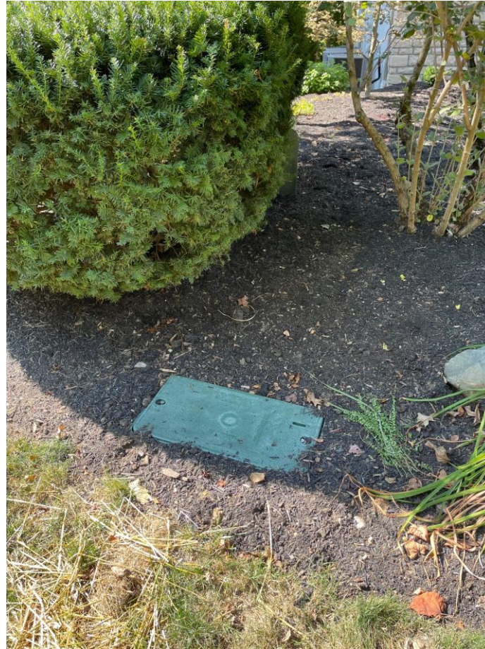
Final installed fiber optic pull boxes
