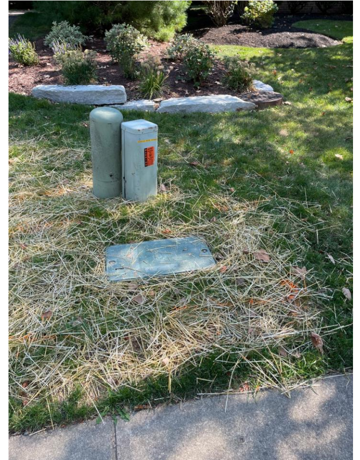
Final installed fiber optic pull boxes
