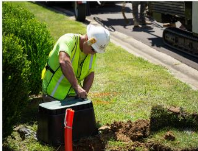
Placing pull box
