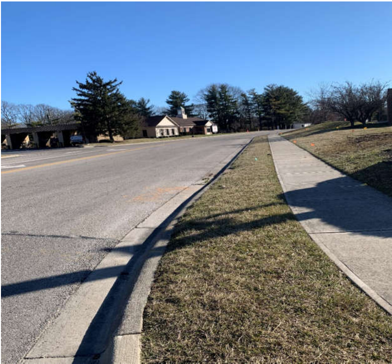
PHOTO 11: View to the south along Corbins Mill Dr.
