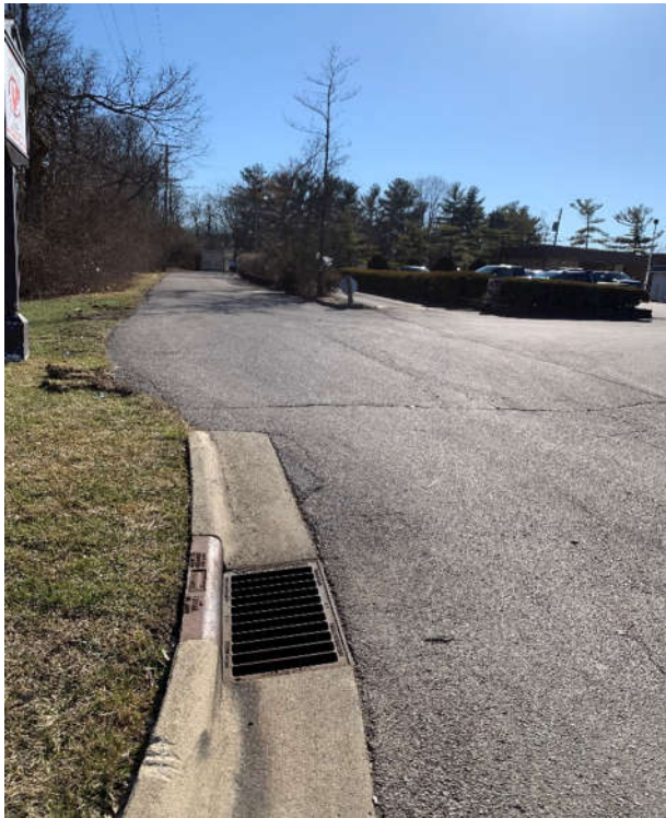
PHOTO 5: View of eastern driveway looking south from sidewalk.
