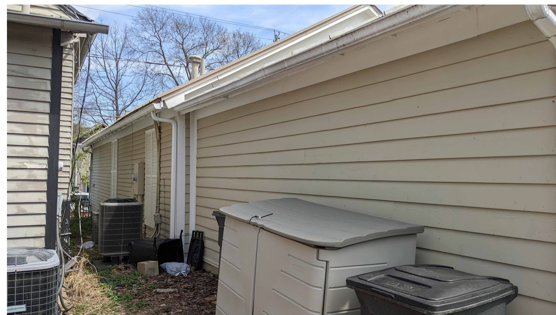
LOOKING EAST FROM EXISTING PARKING LOT TOWARD NORTH BUILDING FACADE
