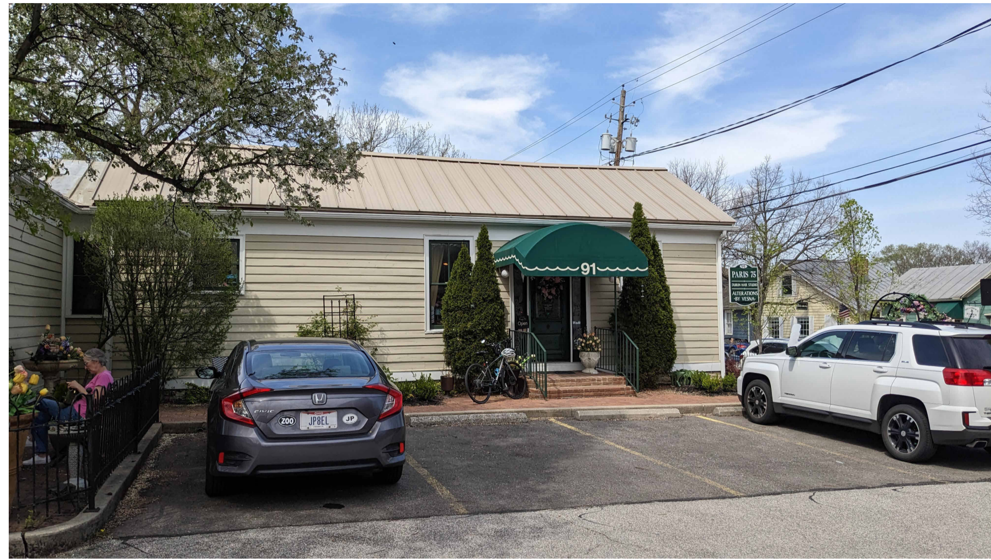
LOOKING NORTH FROM PINNEY HILL LANE TOWARD SOUTH BUILDING FACADE; METAL AND FABRIC AWNING PICTURED TO BE REMOVED
