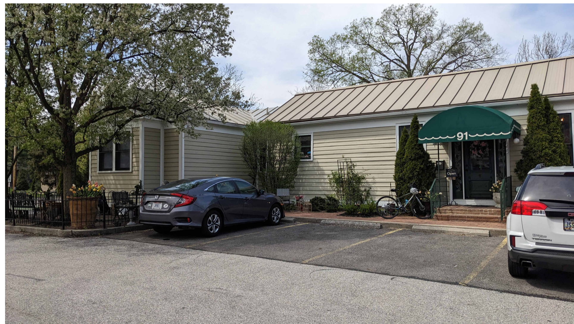
LOOKING NORTH WEST FROM PINNEY HILL LANE TOWARD SOUTH AND EAST BUILDING FACADES; METAL AND FABRIC AWNING PICTURED TO BE REMOVED
