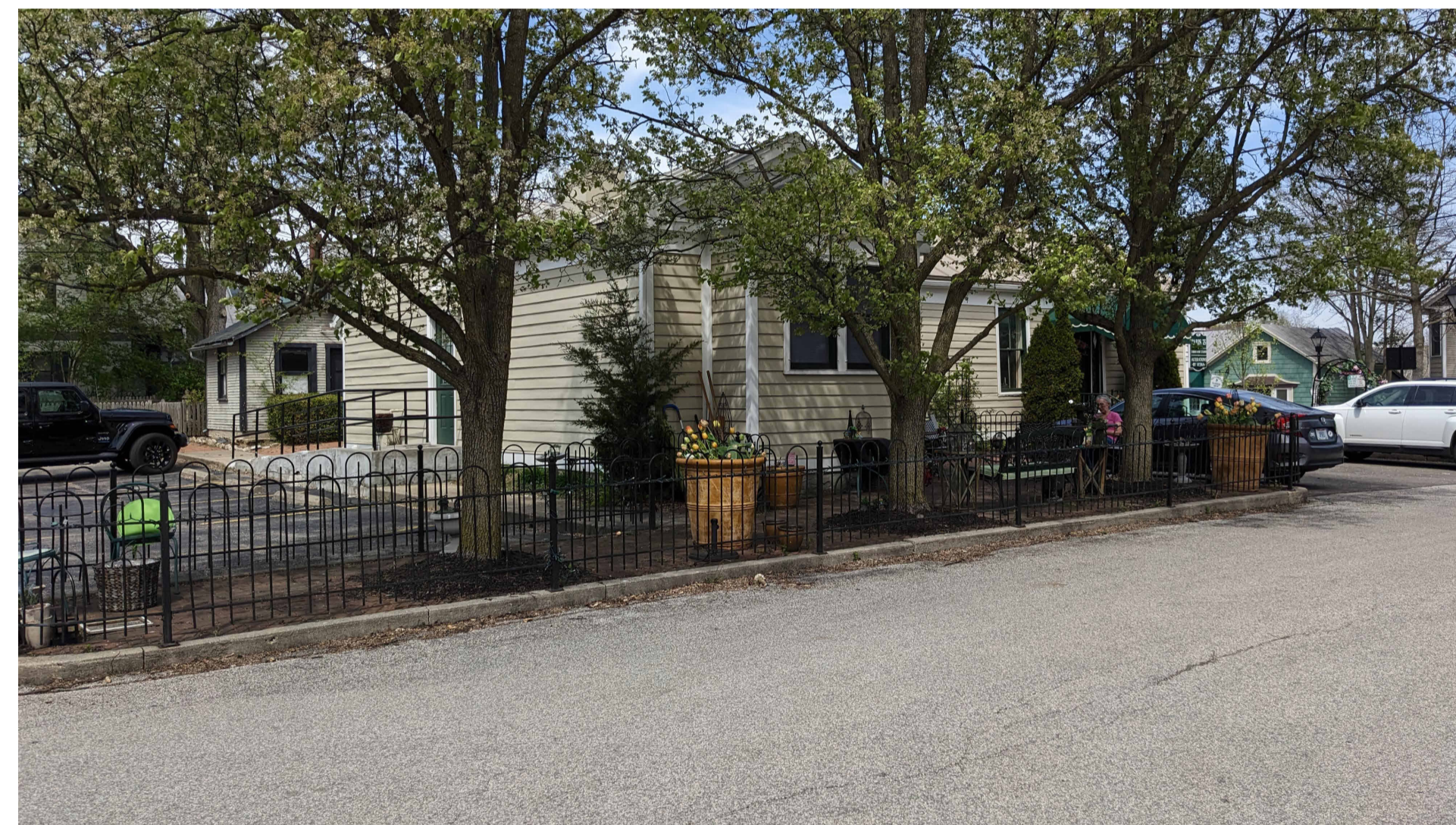
LOOKING NORTH EAST FROM PINNEY HILL LANE TOWARD SOUTH AND WEST BUILDING FACADES AND EXISTING PATIO
