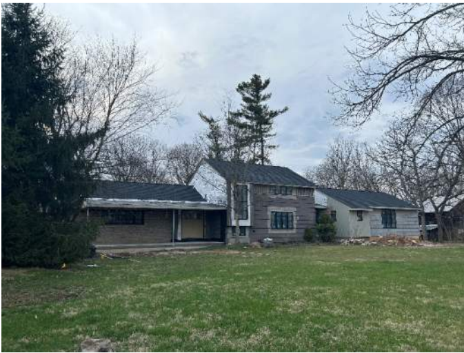
Front porch added to the ranch portion of home in Dublin with pitch less than 3:12.
