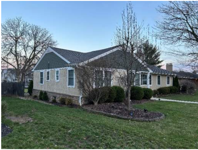
Front Corner Elevation (North-West)
