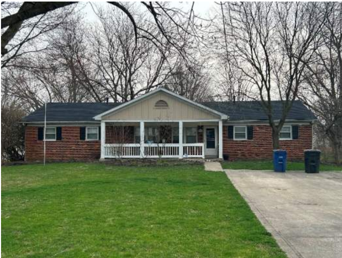
Front porch extension on a ranch home.
