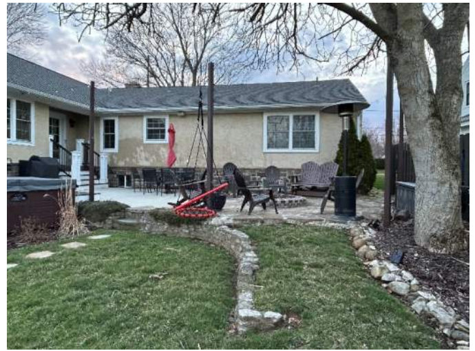
Rear Elevation (East) – Project Addition Area
