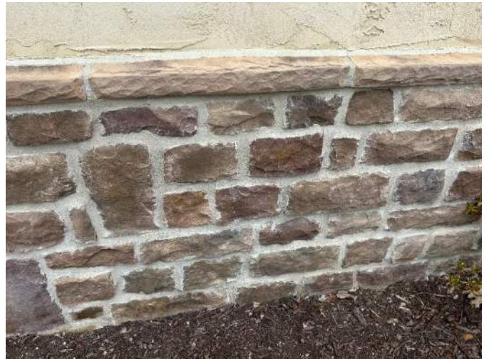
Existing Home - Stone, Sill, Stucco material
