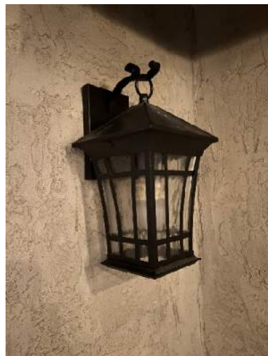
Existing Porch Lighting
