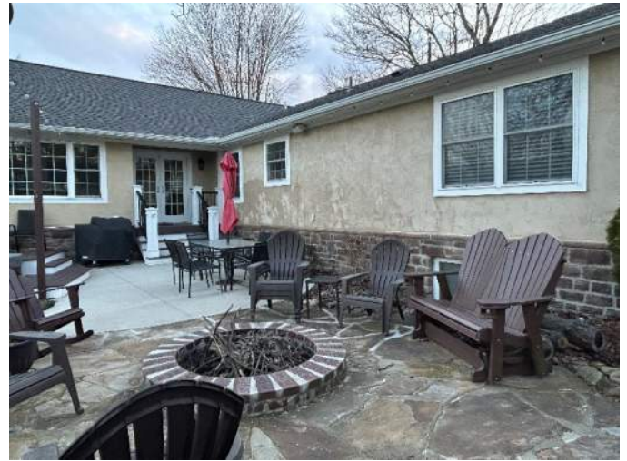
Rear Corner Elevation (North-East)
