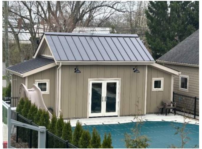
Front Porch Roof – standing seam material example/color from adjacent property
