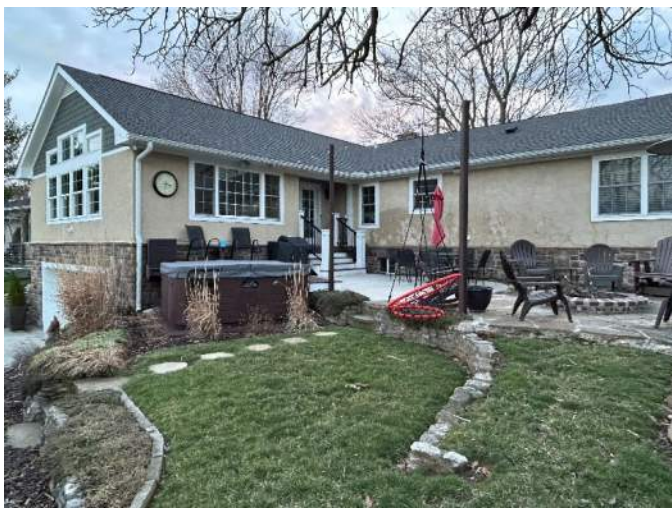
Rear Corner Elevation (North-East)
