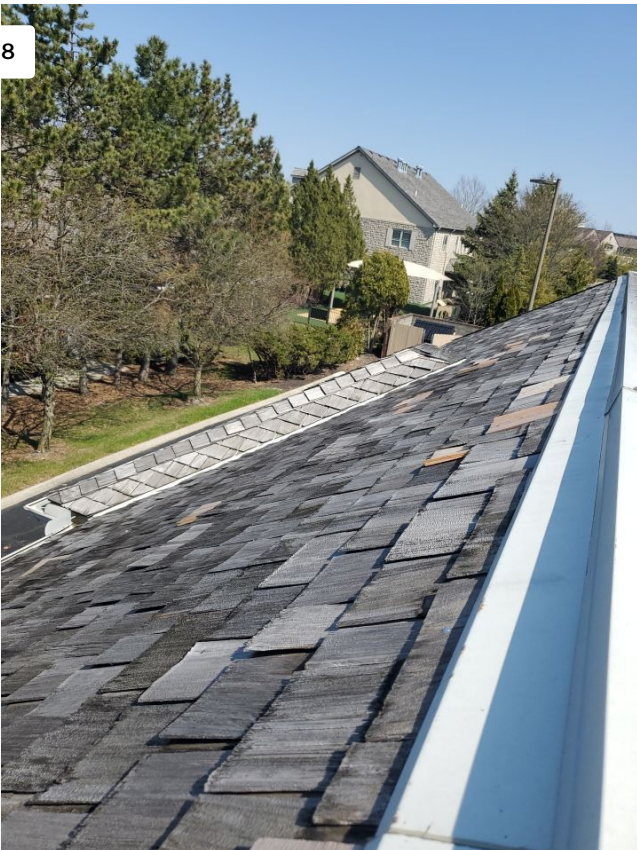
Project: Donato's Pizzeria LLC / 2211-1250931-102 Date: 3/30/2023, 2:19pm Creator: Travis Waggoner
