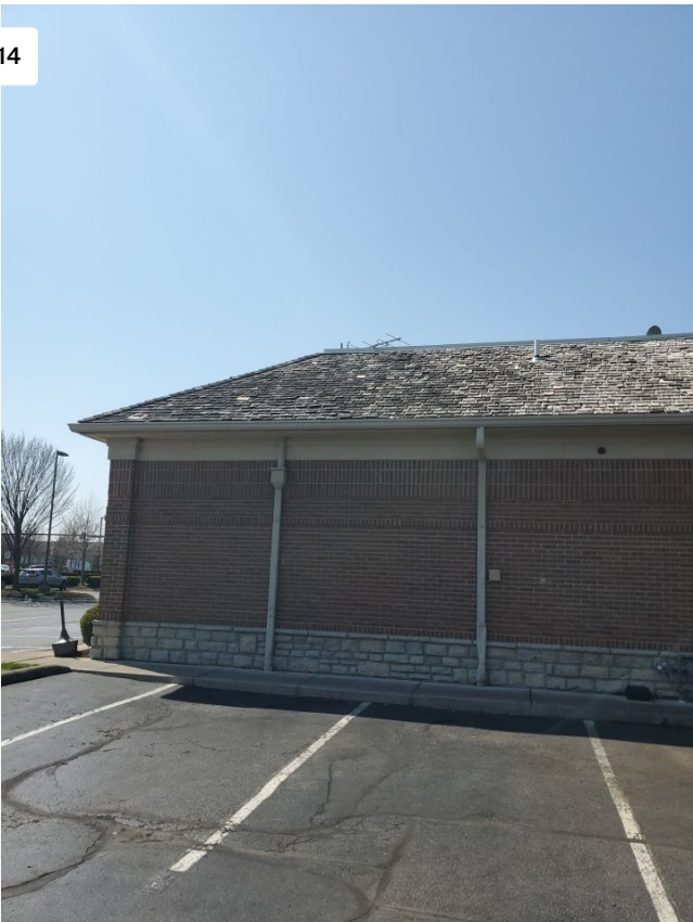
Project: Donato's Pizzeria LLC / 2211-1250931-102 Date: 3/30/2023, 2:30pm Creator: Travis Waggoner
