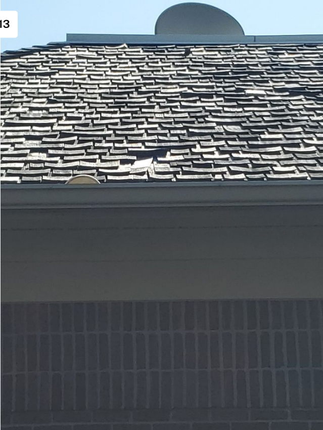
Project: Donato's Pizzeria LLC / 2211-1250931-102 Date: 3/30/2023, 2:29pm Creator: Travis Waggoner
