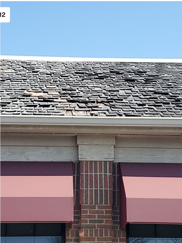
Project: Donato's Pizzeria LLC / 2211-1250931-102 Date: 3/30/2023, 2:28pm Creator: Travis Waggoner
