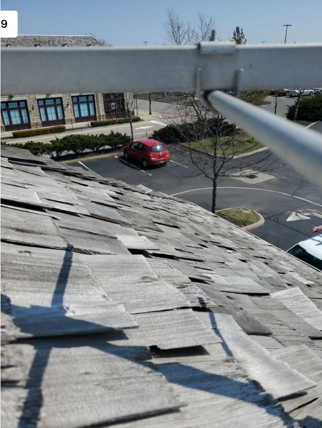
Project: Donato's Pizzeria LLC / 2211-1250931-102 Date: 3/30/2023, 2:20pm Creator: Travis Waggoner
