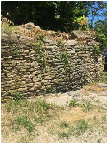
Retaining Wall Buldge at Mid-Height
