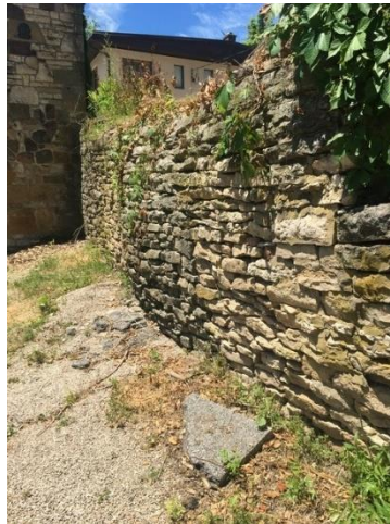
Retaining Wall Buldge at Mid-Height
