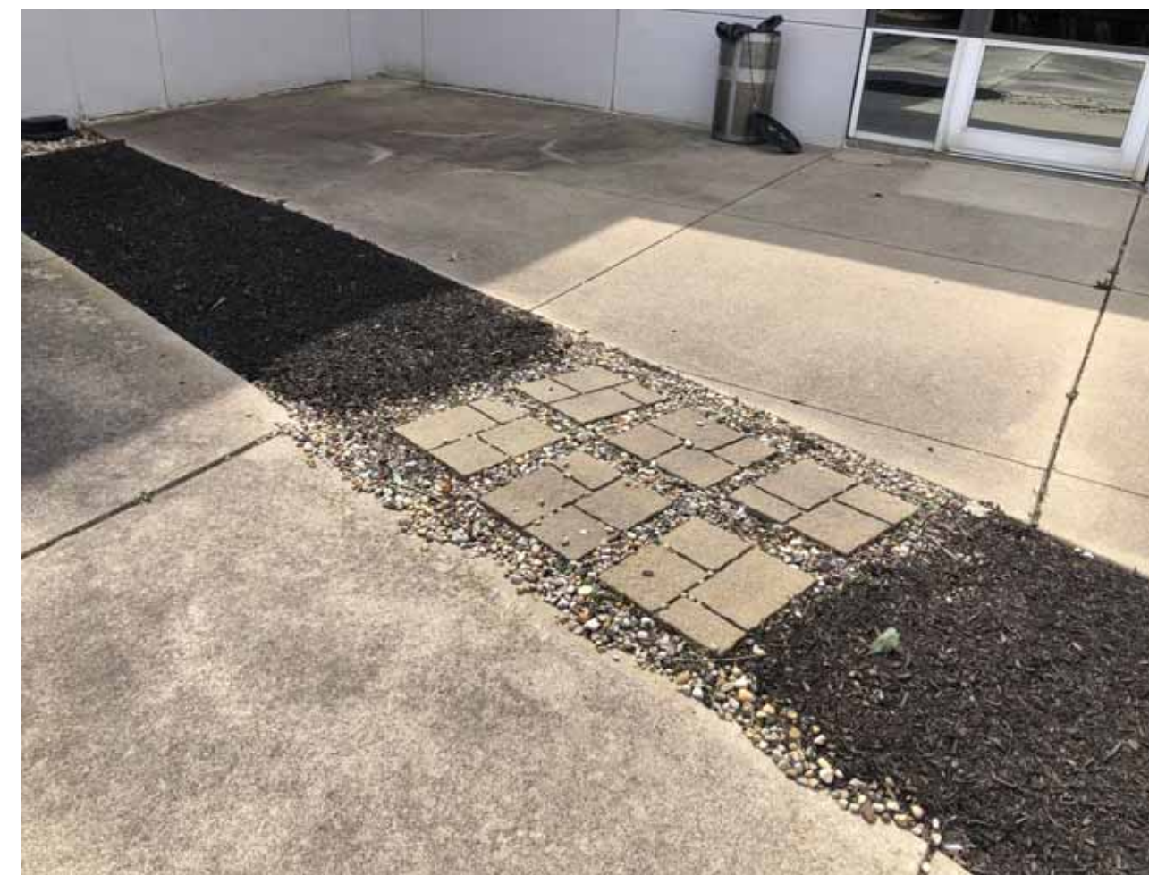
EXISTING SITE PHOTO SHOWING CONCRETE UNIT PAVERS TO BE REUSED IN SAME LOCATION AND PATTERN LAYOUT DURING CONSTRUCTION.
