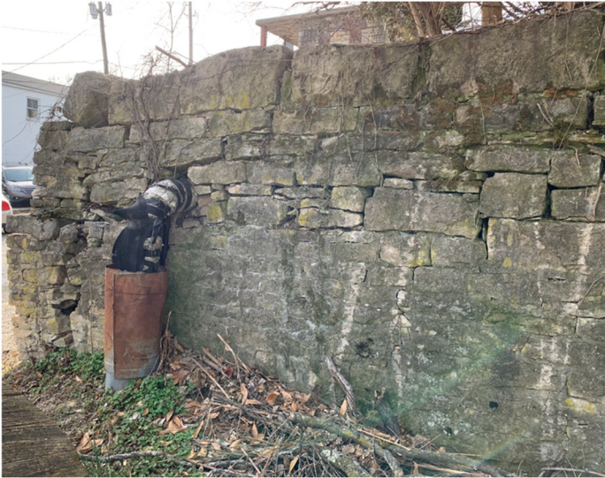
5) East wall detail, looking southwest (February 2023).
