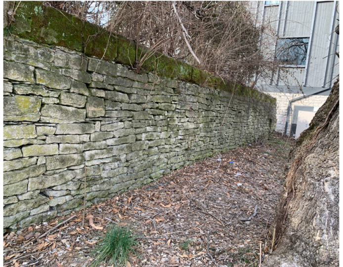
8) East wall detail, looking north-northwest (February 2023).
