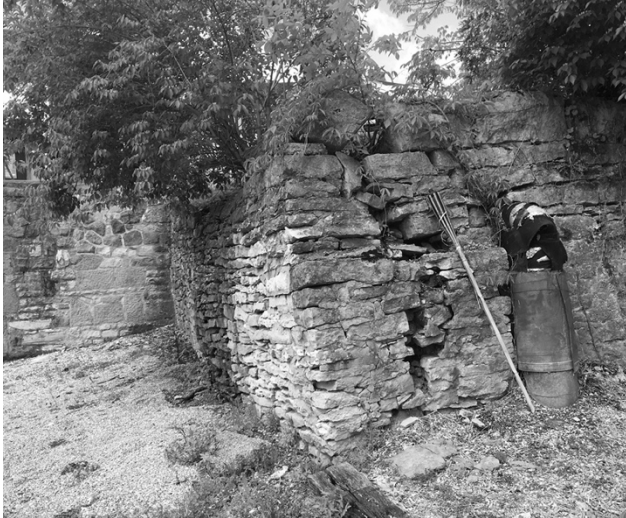
1) Southeast corner of wall, looking west (May 2021).
