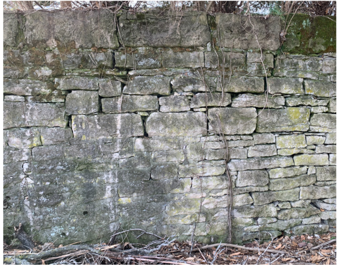
6) East wall detail, looking west (February 2023).
