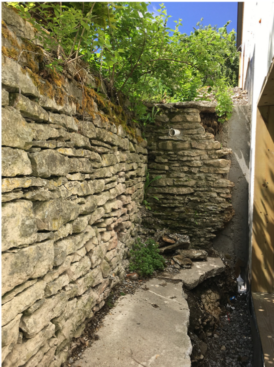
3) North end of wall, facing West (May 2021).
