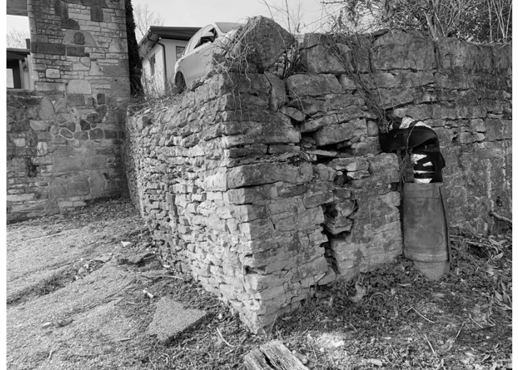
2) Southeast corner of wall, looking west (February 2023).
