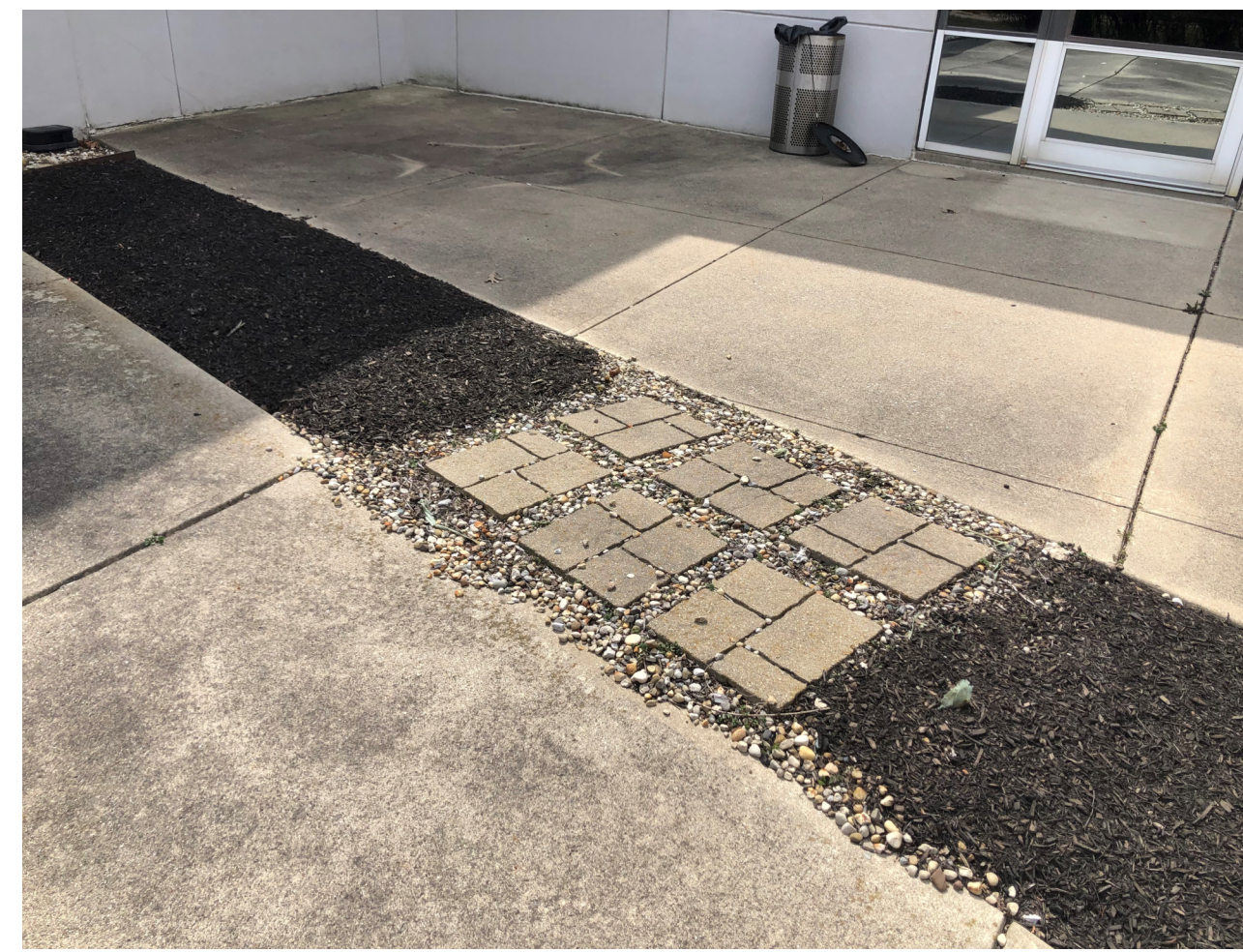
EXISTING SITE PHOTO SHOWING CONCRETE UNIT PAVERS TO BE REUSED IN SAME LOCATION AND PATTERN LAYOUT DURING CONSTRUCTION.
