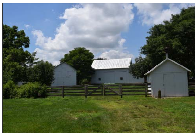
6659 Coffman Rd, outbuildings, looking west
