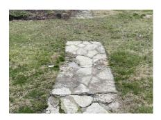
The project also proposes to re-mortar the step leading to the entry on the south façade of the building. The step currently has large gaps where the mortar has disintegrated with time and needs to be repaired for both the safety of visitors and the aesthetics of the Homestead. This activity is determined to be normal maintenance so is not a part of this review.
