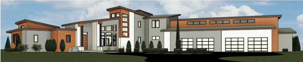
Front Façade (South-facing)
