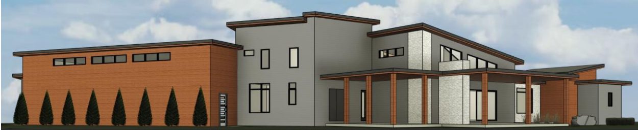
Rear Façade (North-facing)
