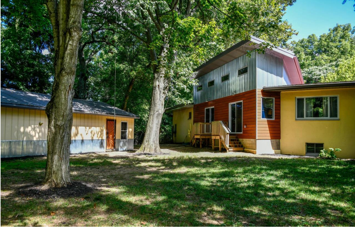
Example 5 (6721 Dublin Road, Previous Dwelling & Structure)
