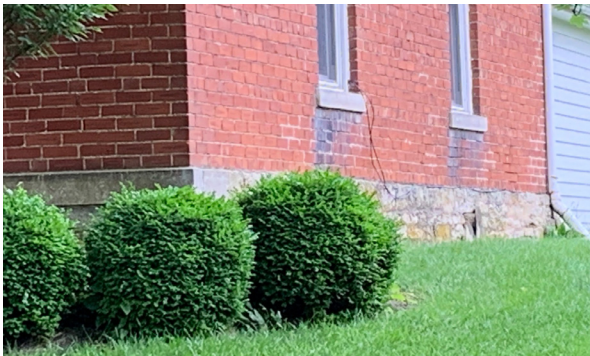
Original stone foundation, 167 South High Street
