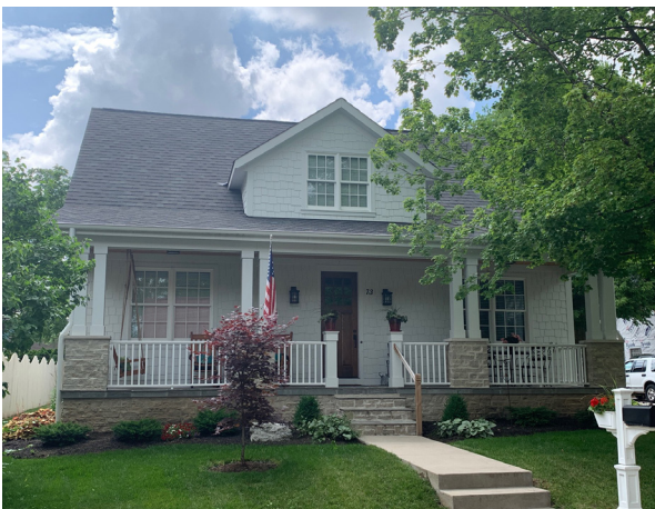
Finished foundation, 73 South Riverview Street
