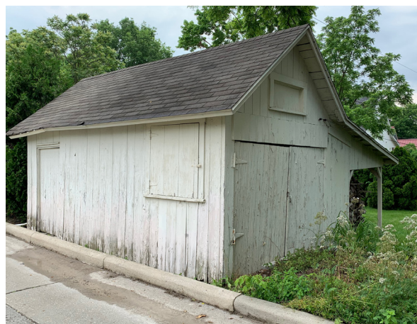
Historic outbuilding, 83 South Riverview Street
