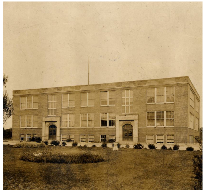
The Washington Township Centralized School at 150 West Bridge Street was built in 1919 in the Art Deco style. Elements of the style include the smooth wall surface and decorative concrete panels with stylized or geometric motifs.
