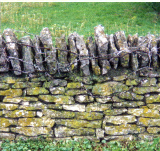
1900s Historic Stone Wall, 2000
