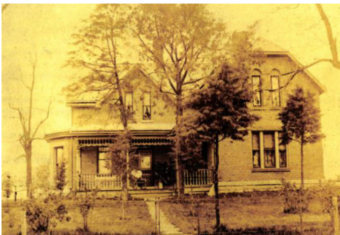
167 South High Street, built in 1897 in the Queen Anne style. Elements of the style include the asymmetrical massing, irregular floor plan, bay windows, decorative gable ends, wrap-around front porch with decorative spindle work, and decorative shingles in the roof.
