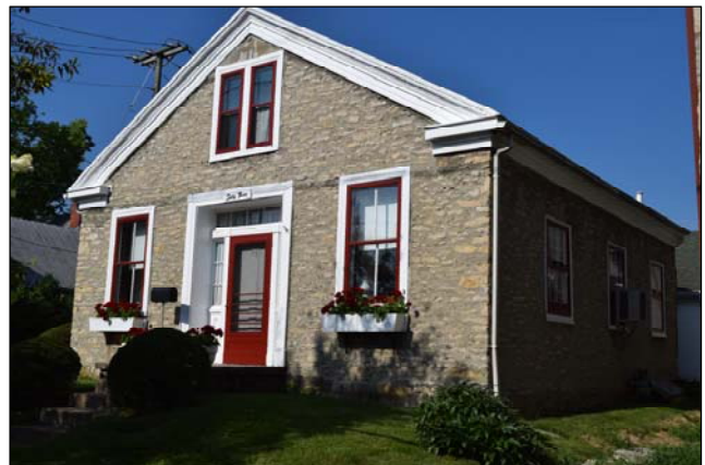
63 S High St, looking southwest
