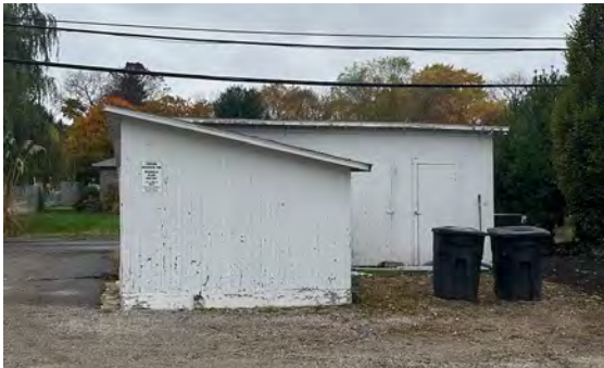
View of the structure from Primary structure:
