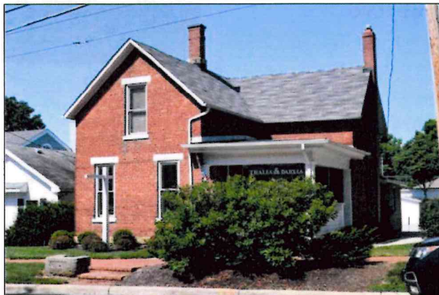
119 S High St, looking southwest
