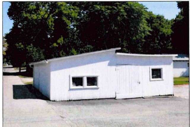
119 S High St, storage building, looking northeast
