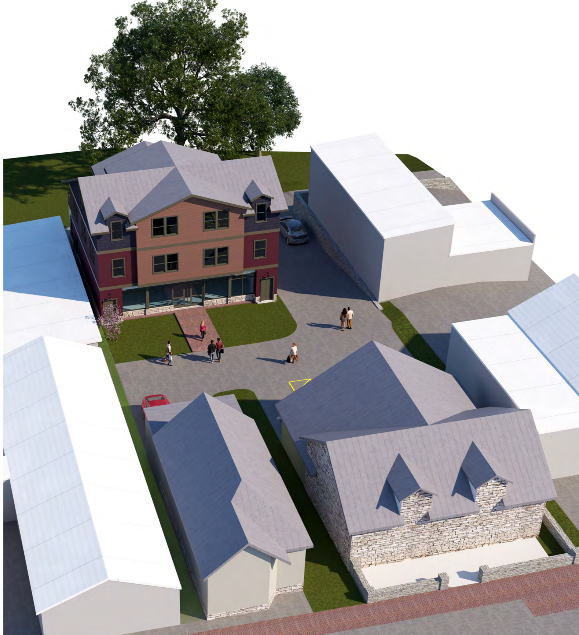
24. Aerial view from the West
