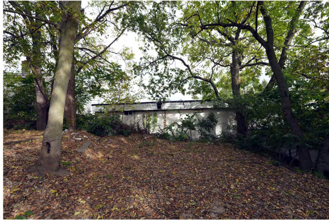
View to the North
