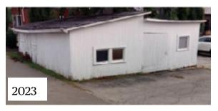
The condition of this utility shed is poor and most of the materials would need to be replaced rather than repaired. Most of the trim work and window detail is uneven and out of alignment. Doors are made of pieces of siding and secured with padlocks. There appears to have been a large opening on the Mill Street side that has been sealed shut with painted plywood.
