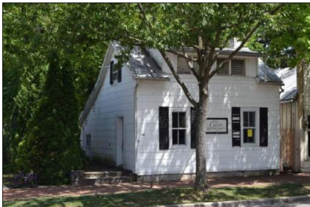
30 S High St, looking southeast
