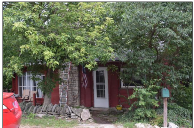
62 N Riverview St, looking northeast
