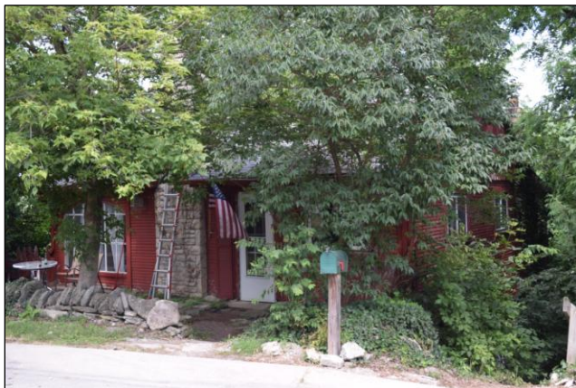
62 N Riverview St, looking southeast
