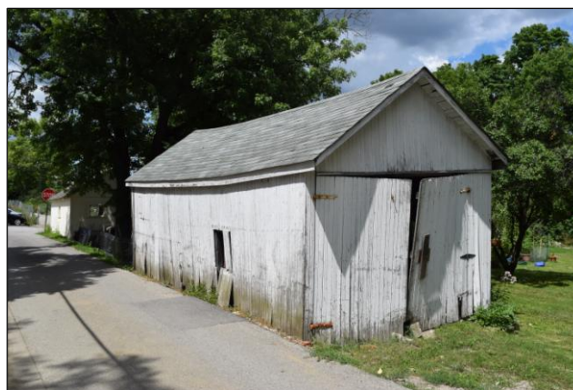
45 N Riverview St, ancillary structure, looking northeast
