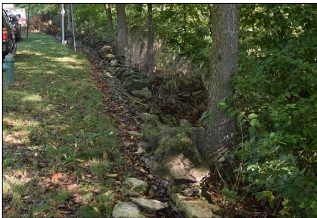
Overview of wall, looking north
