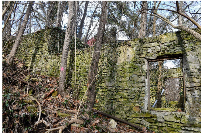
Foundation Remains (South Wall)
