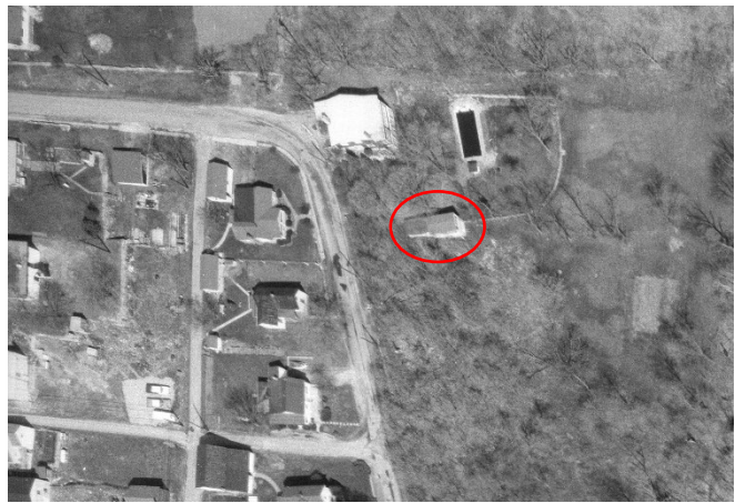
Structure Photo (1963 ODOT Aerial)
