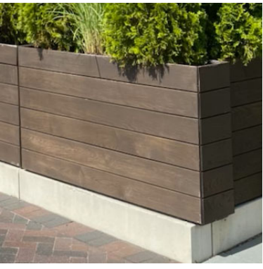
NEW WOOD PANELED PLANTERS (MATCH EXISTING PLANTERS) 5" L X 1' W X 3' H
