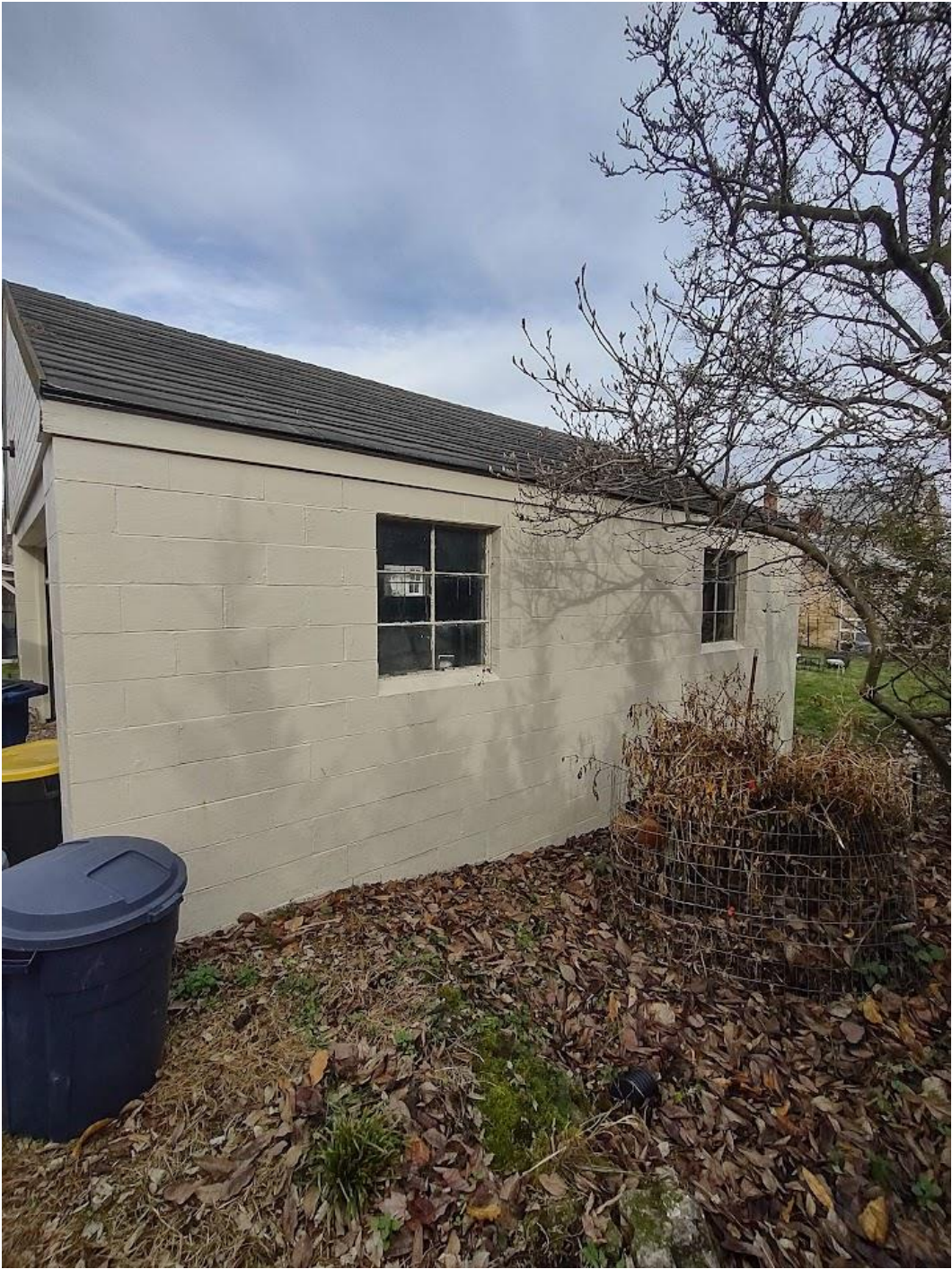
South building side
