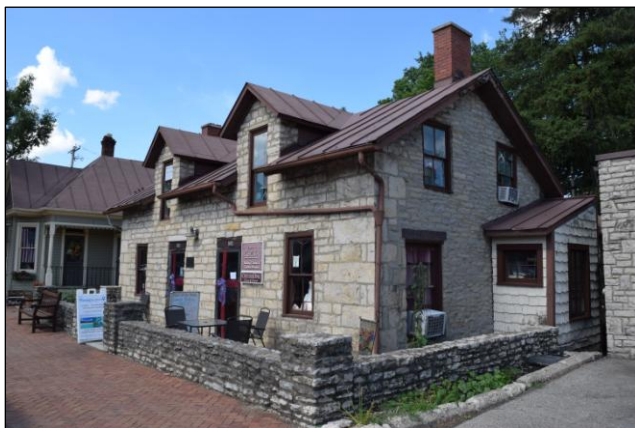
16 N High St, looking northeast
