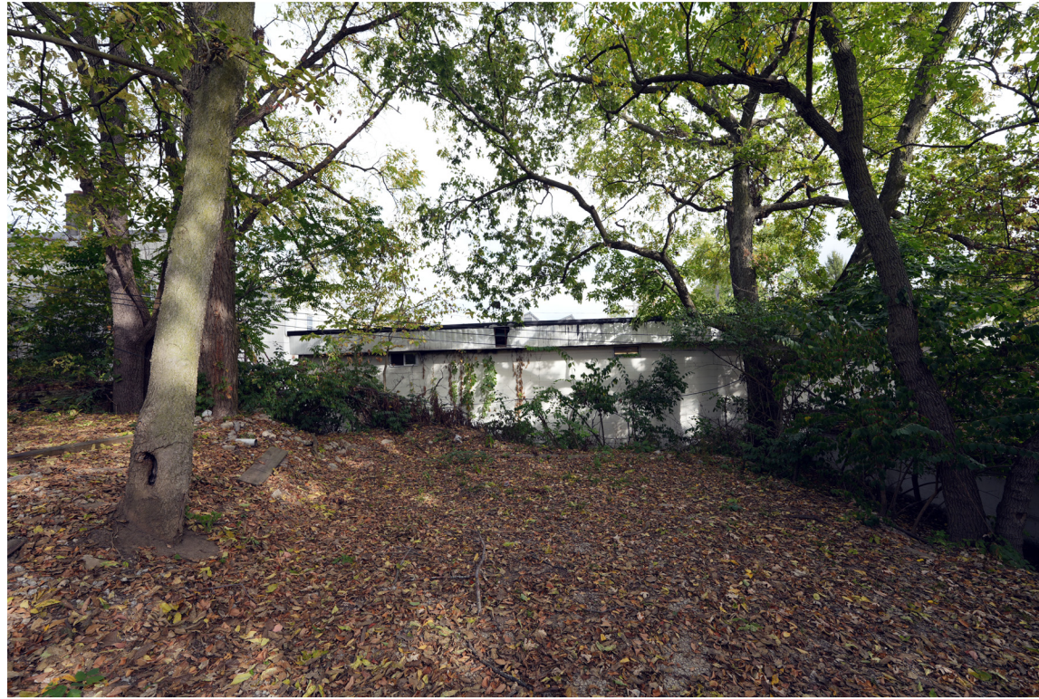
View to the North
