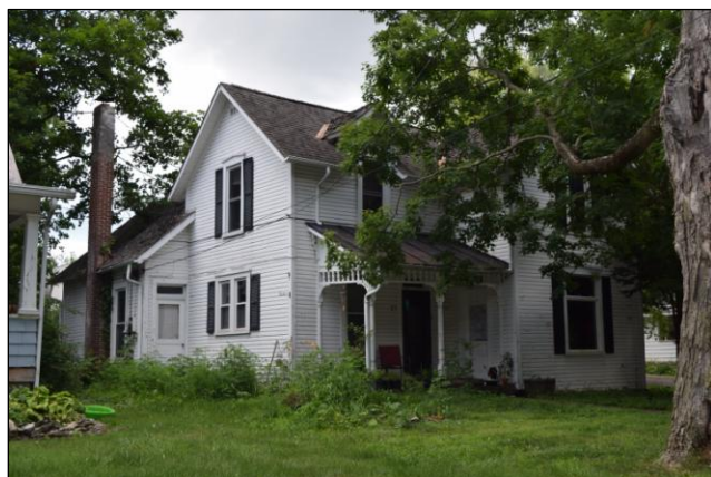
27 N Riverview St, looking northwest
