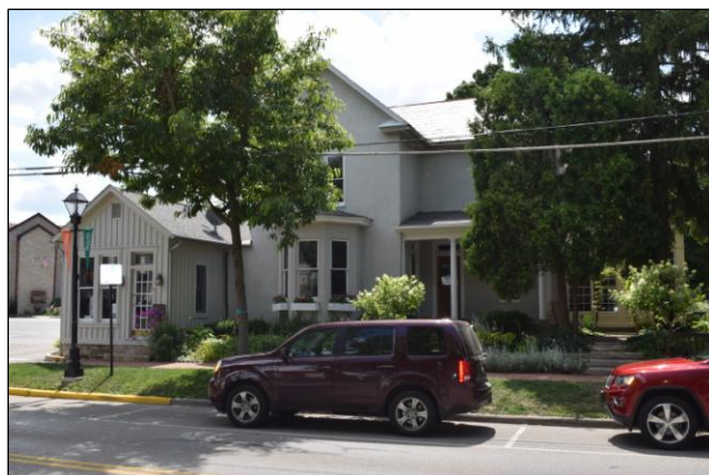
35 S High St, looking southwest
