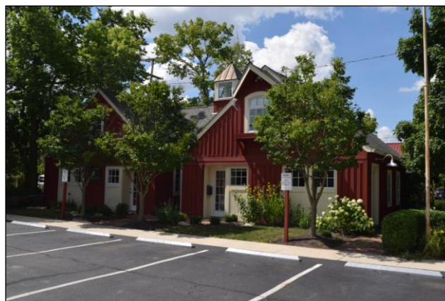
35 S High St, rear modern building, looking northwest
