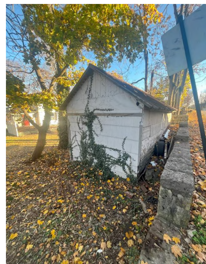
OUT BUILDING NW CORNER OF LOT
