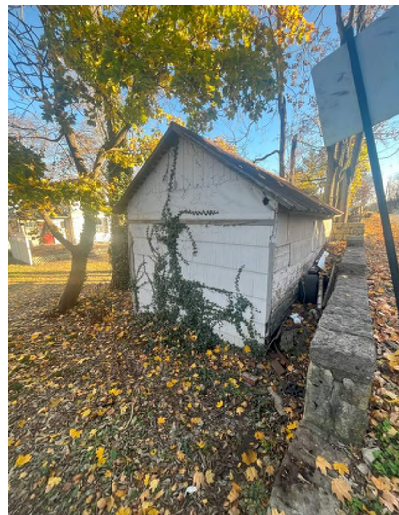
OUT BUILDING NW CORNER OF LOT
