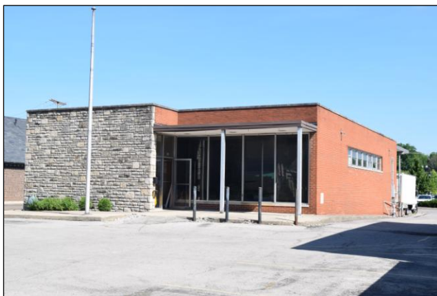
38 W Bridge St, looking northwest
