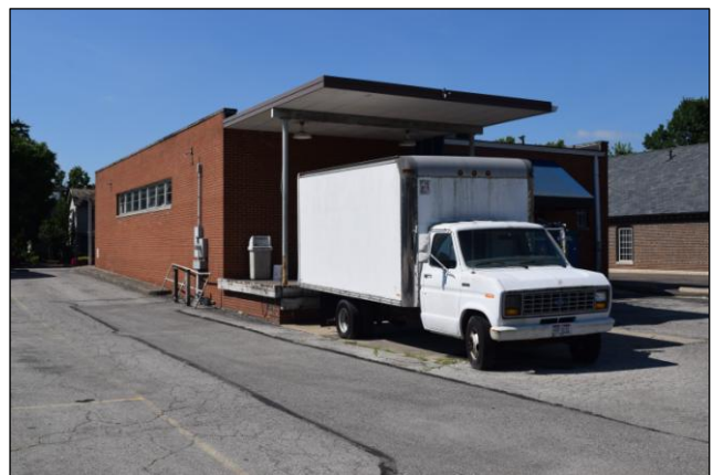
38 W Bridge St, looking southeast
