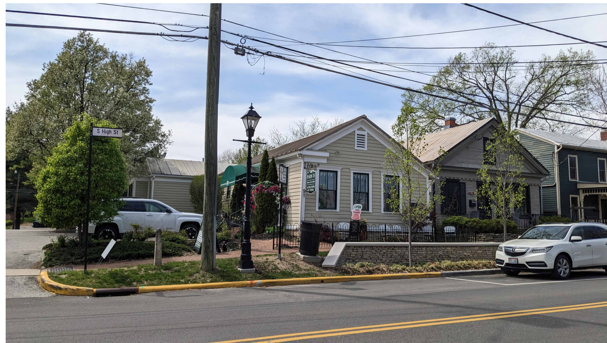
LOOKING WEST FROM EAST SIDEWALK ON S. HIGH STREET TOWARD EAST BUILDING FACADE
