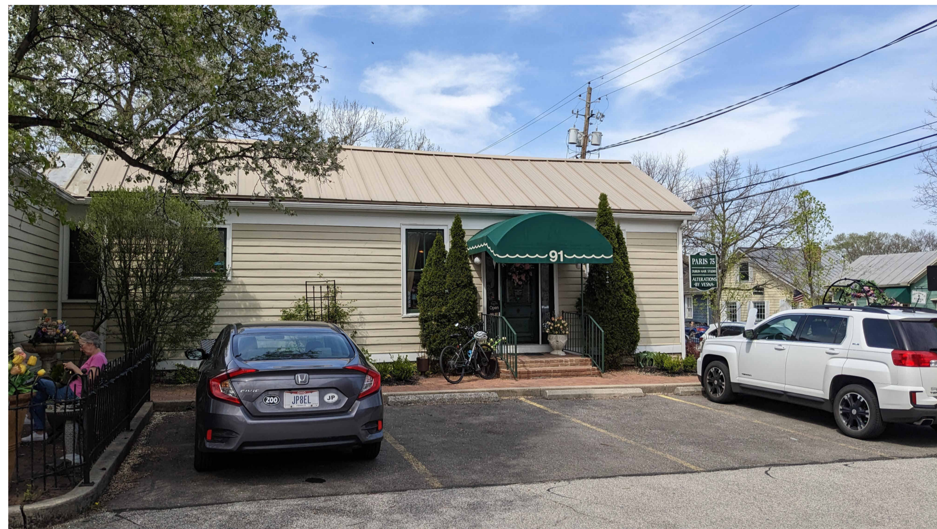
LOOKING NORTH FROM PINNEY HILL LANE TOWARD SOUTH BUILDING FACADE; METAL AND FABRIC AWNING PICTURED TO BE REMOVED
