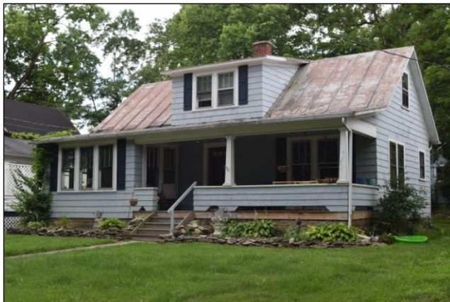
17 N Riverview St, looking southwest
