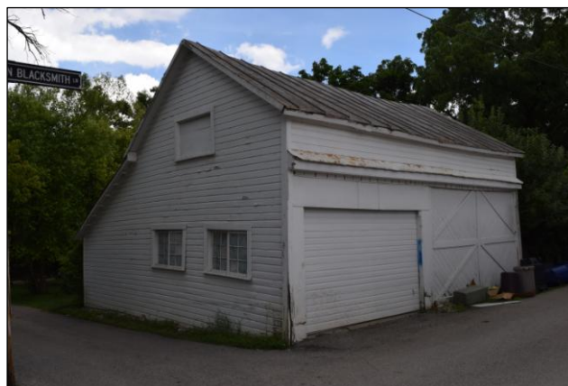
27 N Riverview St, carriage barn, looking southeast
