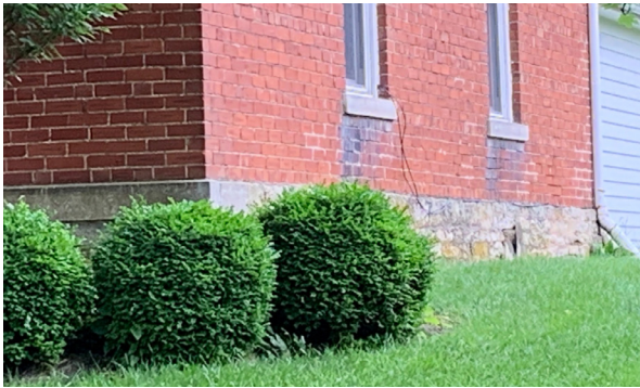
Original stone foundation, 167 South High Street
