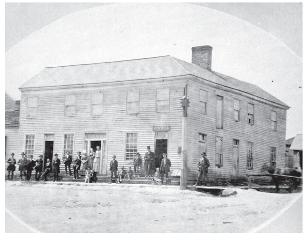
Coffman's Corner, SW Corner - Bridge Street at High Street, 1879
