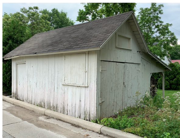
Historic outbuilding, 83 South Riverview Street
