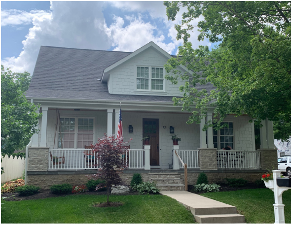
Finished foundation, 73 South Riverview Street
