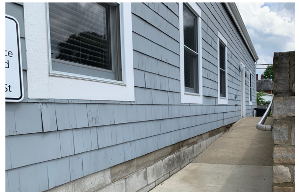
Rear ADA ramp with masonry wall, 129 South High Street
