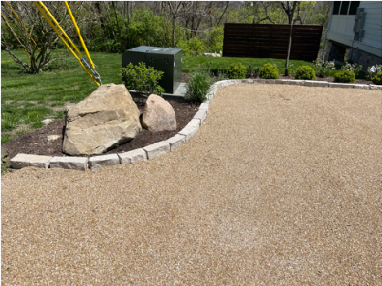
Walkway: Brassfield fines fill
