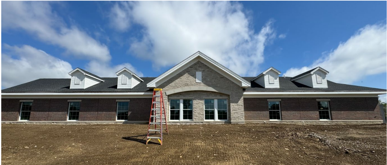
Newly constructed specialty hospital.
